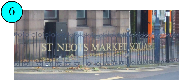
Find the protective unique railings at the cross roads
